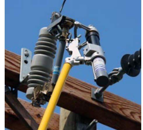
Figure 2 - Attaching the XLT
